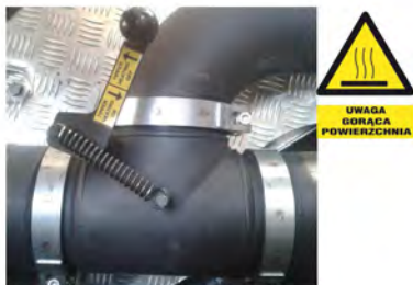
Fig. 36. Exhaust gases distribution valve
